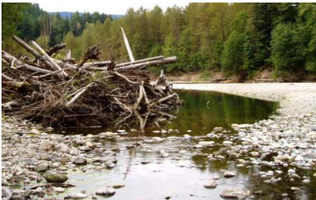
Photograph 1 Natural retention of mobile wood and pool formation at an ELJ on the Stillaguamish River, Washington
