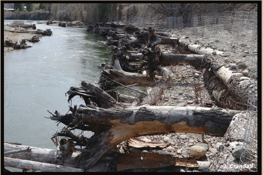
An example of an engineered large wood jam at the Whitefish Island project area south of Winthrop.
